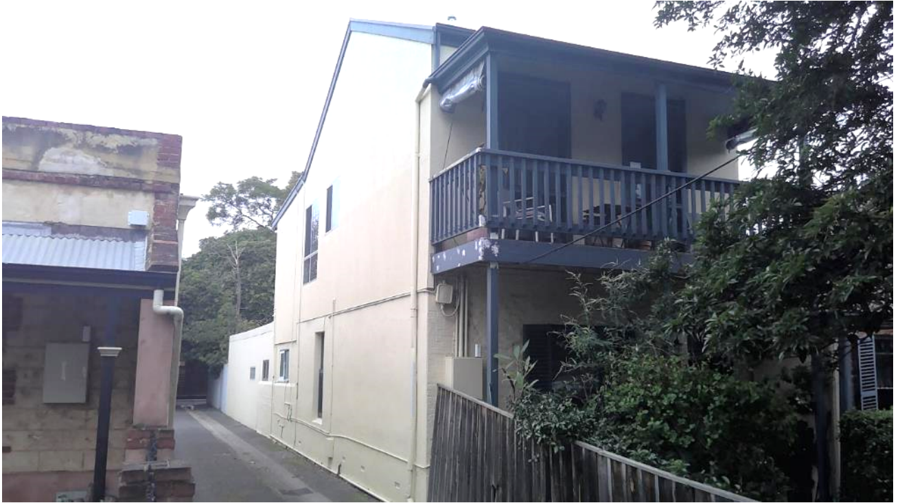
Figure 3.5 – Row cottage adjacent subject site to the east
